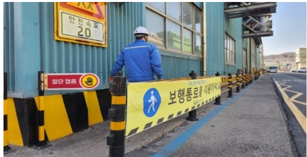
Installing in-house pedestrian pathways to prevent accidents while walking
